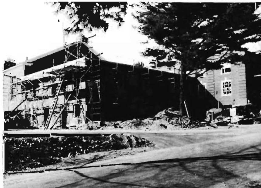
New locker rooms being constructed
