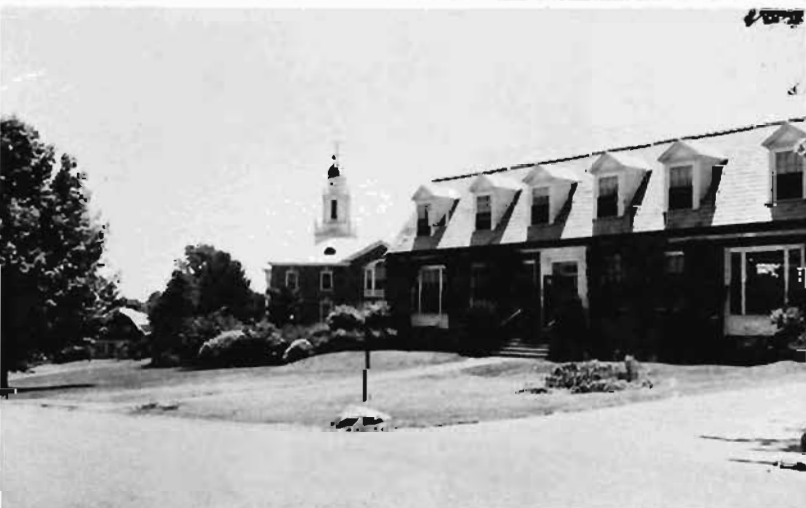
Administration's offices the heart of Babson
