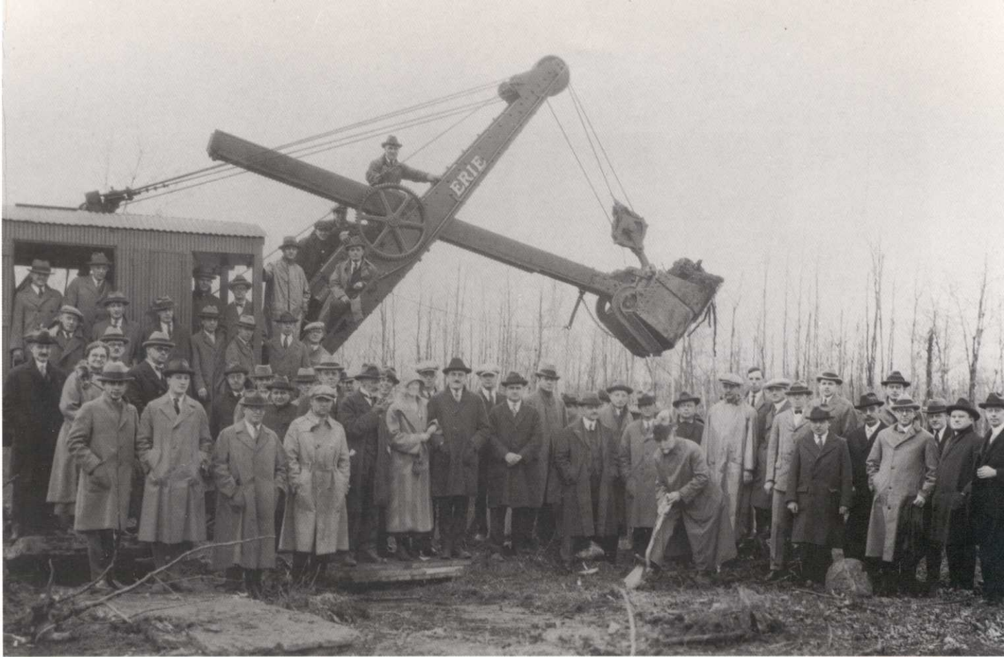
Groundbreaking for the Newton Library in 1938.
