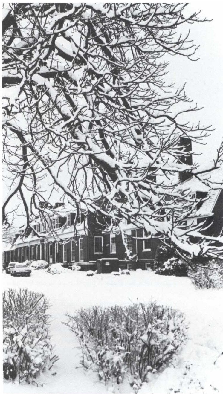
Forest Hall, a residence, was once the Convalescent Home, the property of Boston’s Children’s Hospital. Polio patients used to be sent there to recuperate. Babson Institute bought the building and several other hospital structures in 1959.
